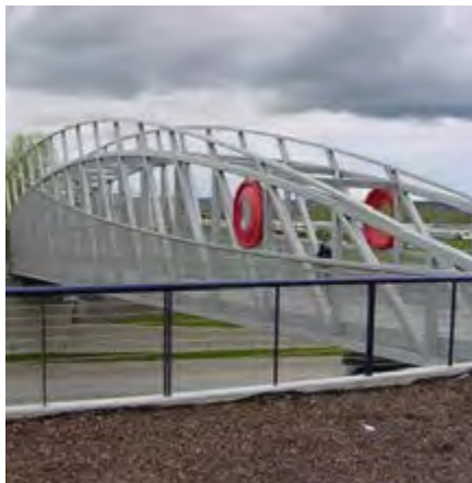
Pedestrian bridge in Portland, OR
