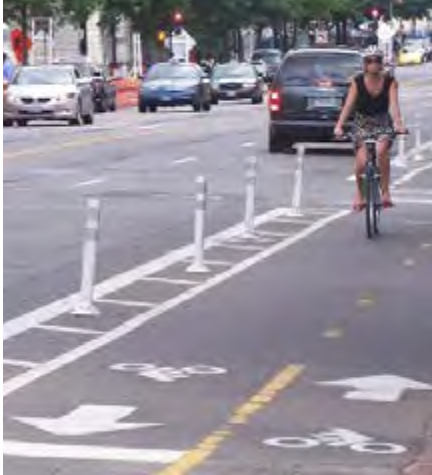
Cycle track with bollard separation
